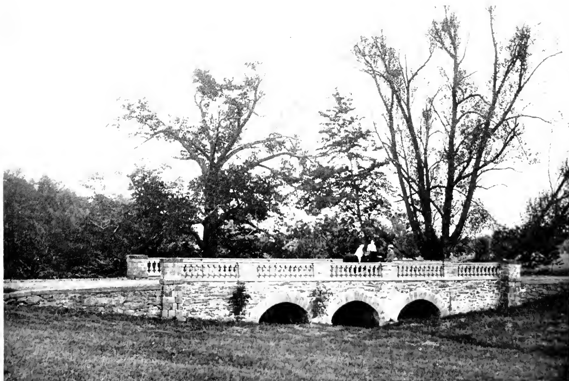
A substantial stone bridge spanning a depression in the driveway of a country estate.
